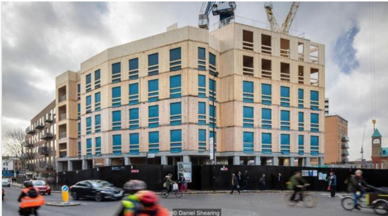
Waugh designed this 10-storey development in Dalston, London. The CLT structure weighs just one fifth of an equivalent concrete building (Credit: Daniel Shearing)
